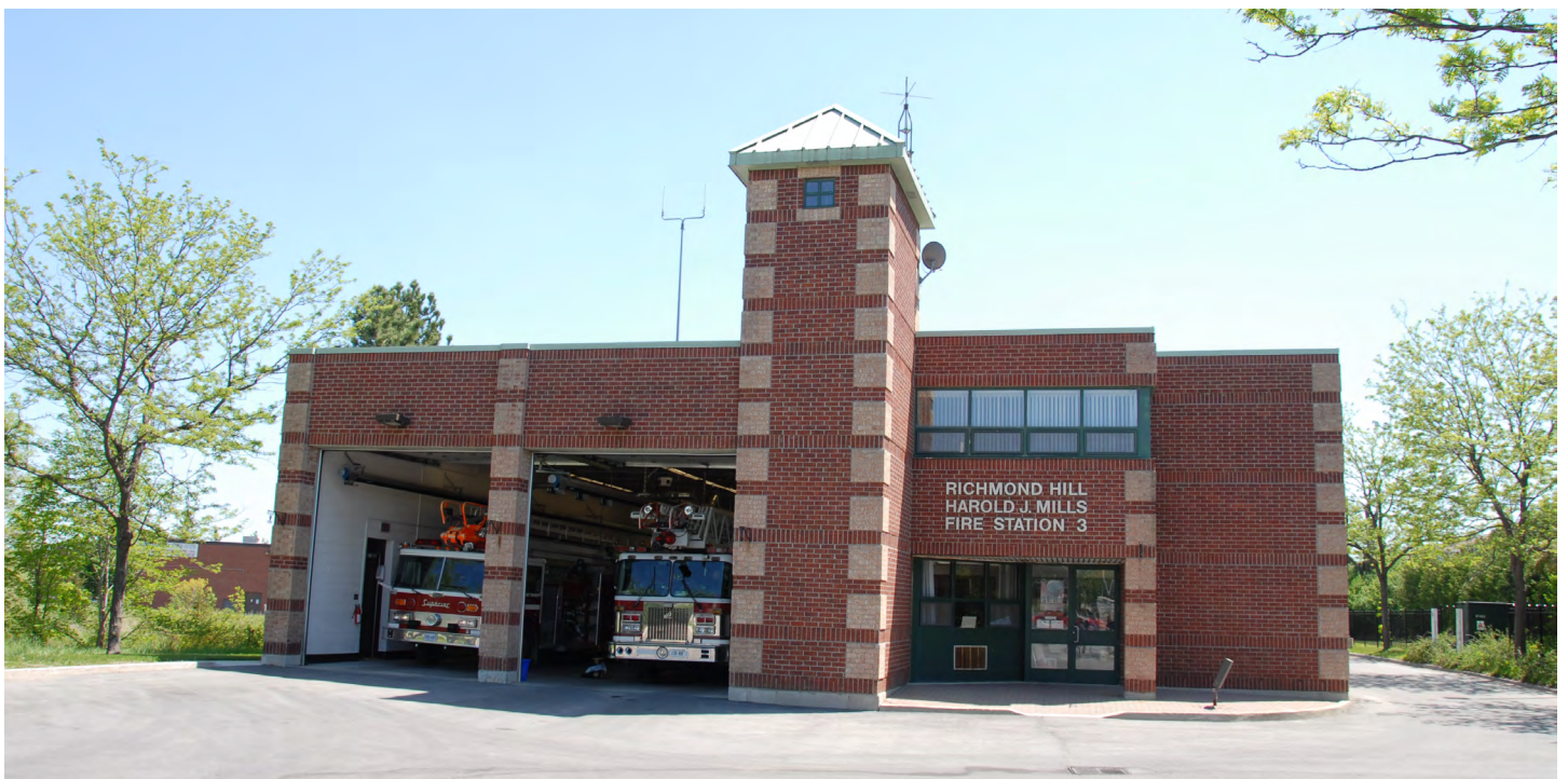
Fire Station 8-3 (Harold J. Mills)
