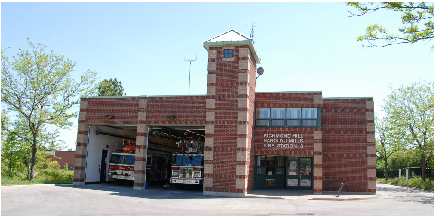
Fire Station 8-3 (Harold J. Mills)
