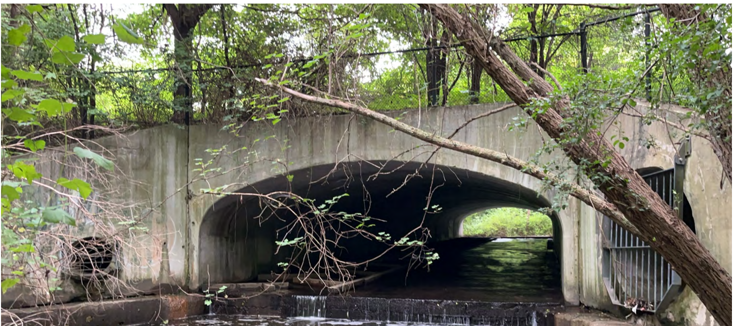
Boake Trail Culvert
