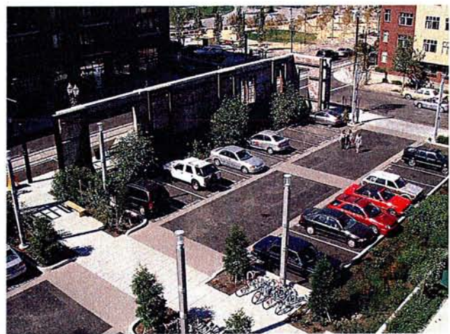
PARKING FACILITY WITH STORMWATER MANAGEMENT IN PORTLAND, OREGON
