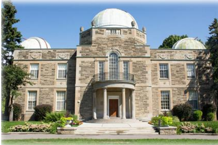
FIGURE 2.3-14 THE DAVID DUNLAP OBSERVATORY IS A NATIONAL HISTORIC SITE LOCATED BETWEEN YONGE STREET AND BAYVIEW AVENUE NORTH OF 16TH AVENUE, BUT WITH LIMITED VISIBILITY FROM THESE ARTERIAL STREETS.
