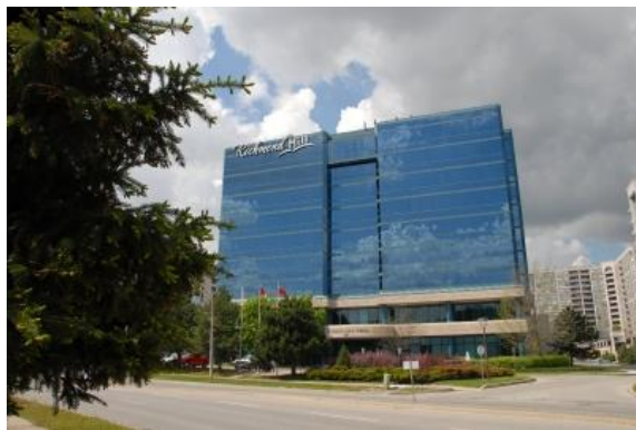
FIGURE 2.3-11 RICHMOND HILL MUNICIPAL OFFICES ARE LOCATED WITHIN THIS CENTRE AMIDST OTHER OFFICE, RETAIL, HOSPITALITY AND RESIDENTIAL DEVELOPMENT
