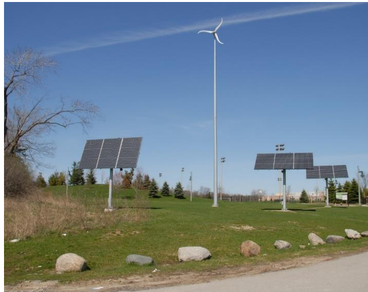
FIGURE 2.5-3 RENEWABLE ENERGY INSTALLATIONS AT RICHMOND GREEN SPORTS CENTRE AND PARK
