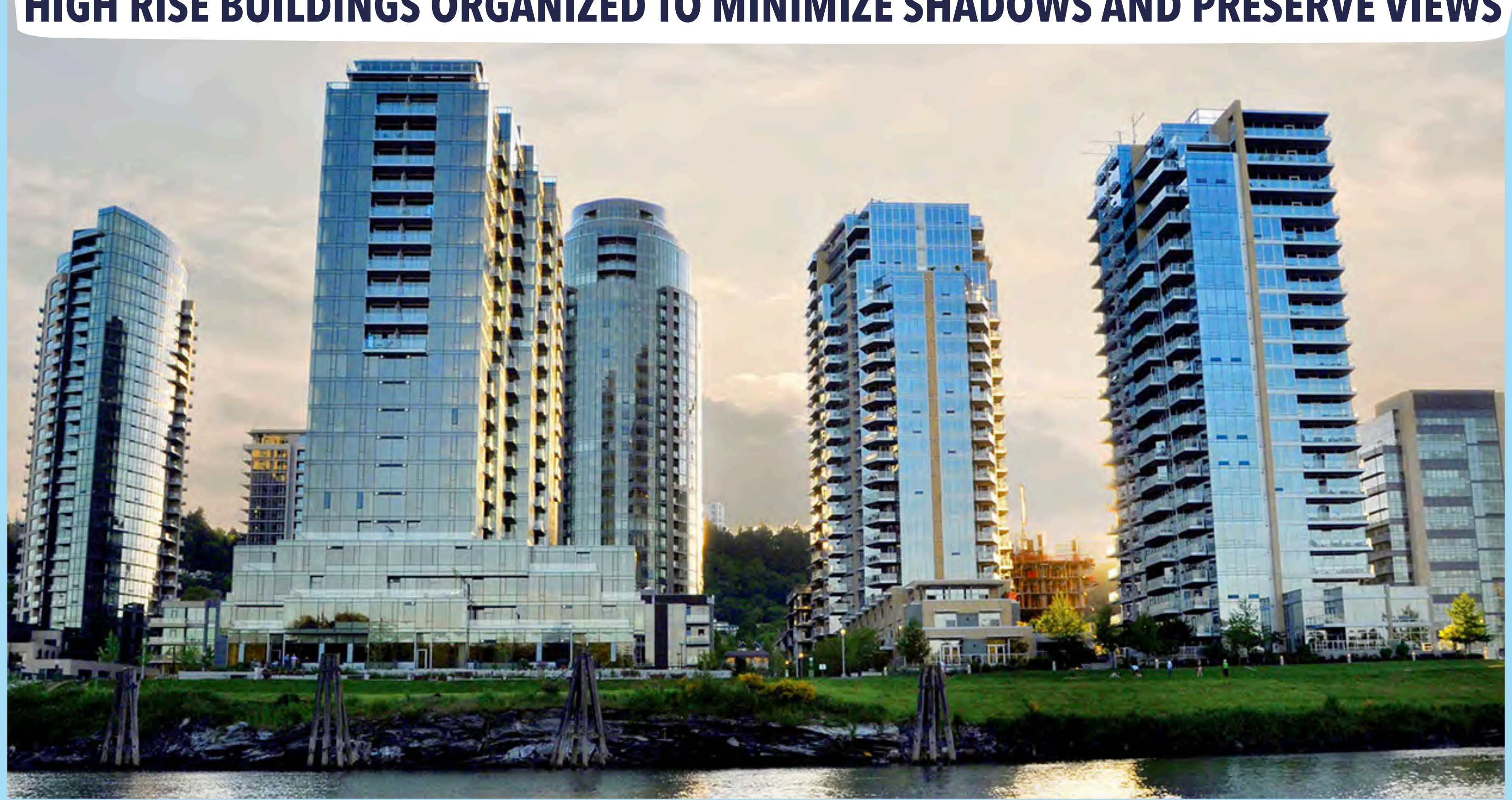
South Waterfront, Portland, USA HIGH RISE BUILDINGS ORGANIZED TO MINIMIZE SHADOWS AND PRESERVE VIEWS
