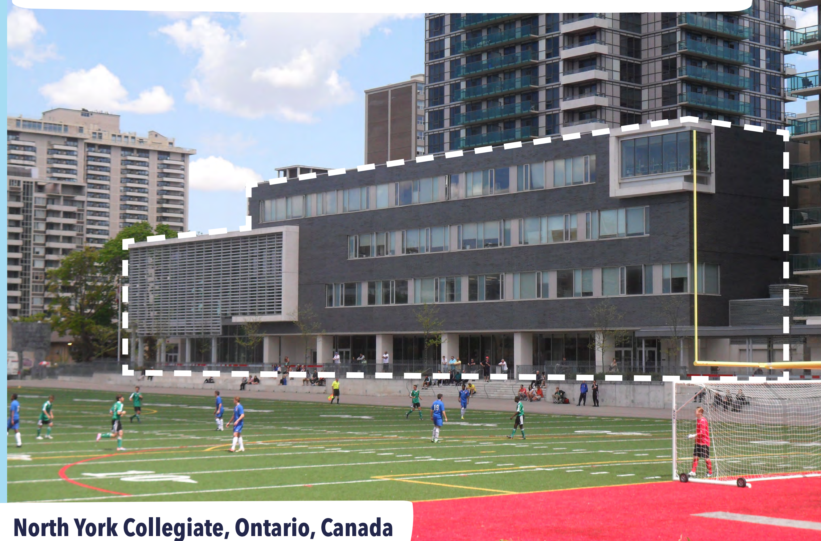
A NEW HIGH SCHOOL INTEGRATED INTO THE BASE OF AN APARTMENT BUILDING
