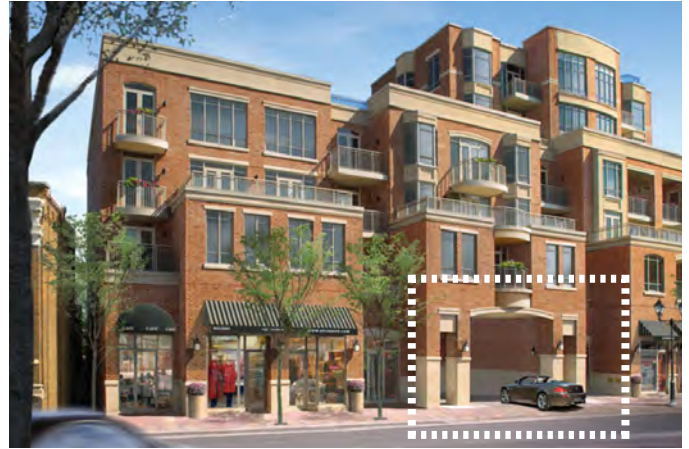
Parking and servicing access from Yonge Street integrated within a mid-rise building fronting Yonge Street, Richmond Hill
