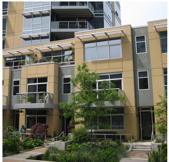
Residential ground floor units in a tall building podium
