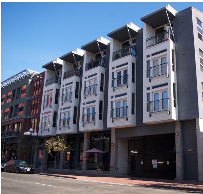
Integrating entrances to underground parking both physically and visually with site and building design and incorporating active at-grade uses helps to animate a streetscape
