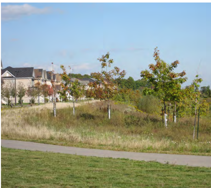
Barrier-free access is provided adjacent this SWM feature
