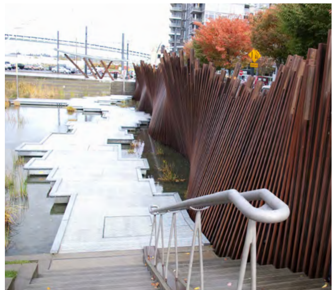
A pedestrian walkway, public art and signage is incorporated into this SWM feature
