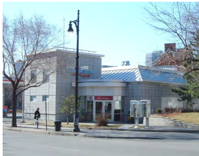
Providing an entrance door from both the pump side and the street is encouraged
