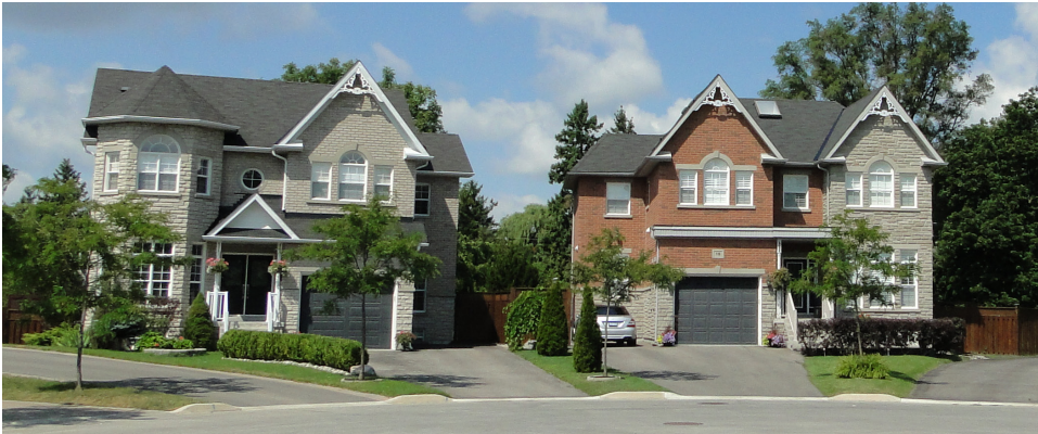
Consistent building forms and styles, height, and massing
