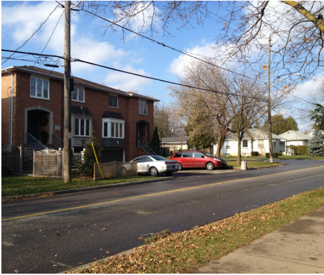
Varied building height and massing
