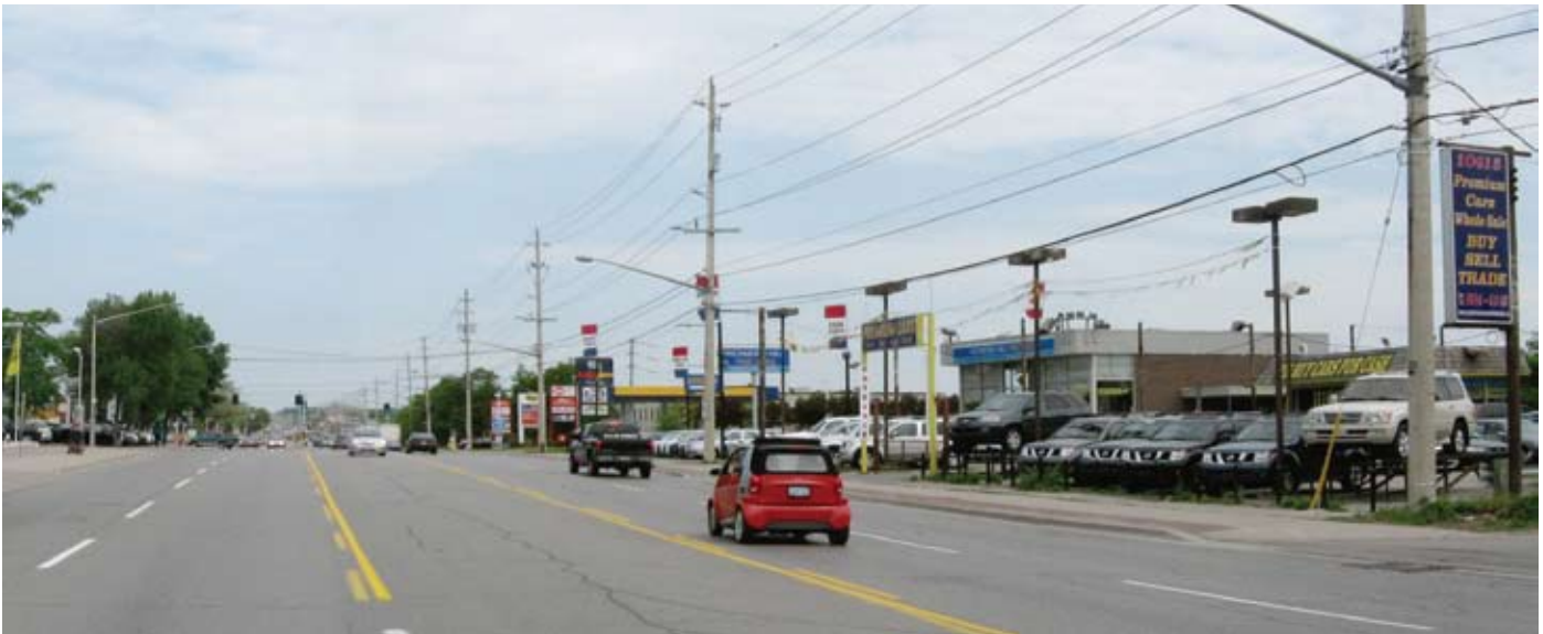
Uptown District: existing conditions
