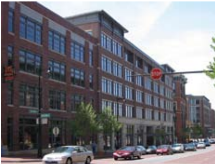
Above: Examples of buildings with a mix of ground related uses that animate the street
