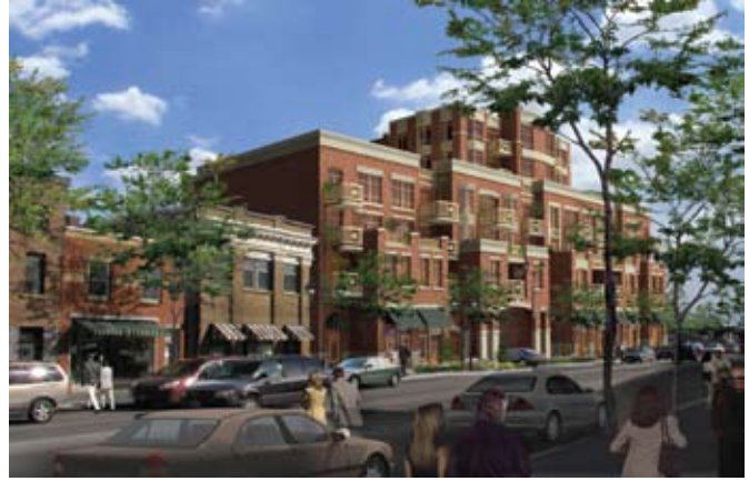
10097 and 10101 Yonge Street rendering with grade-related uses, base building and step back to upper storeys
