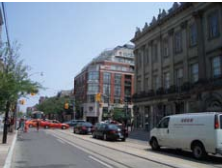
Examples of buildings with contextually appropriate height and massing
