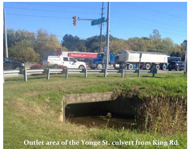
Outlet area of the Yonge St. culvert, looking west
