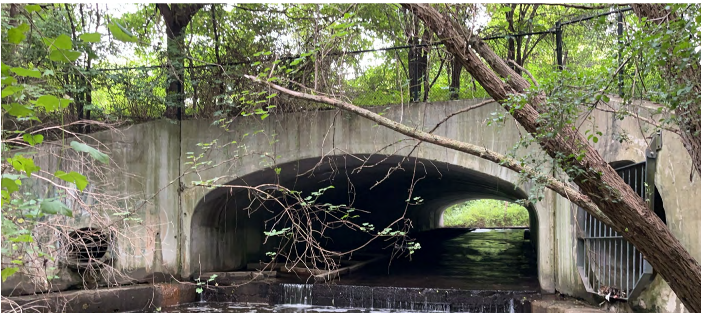
Boake Trail Culvert
