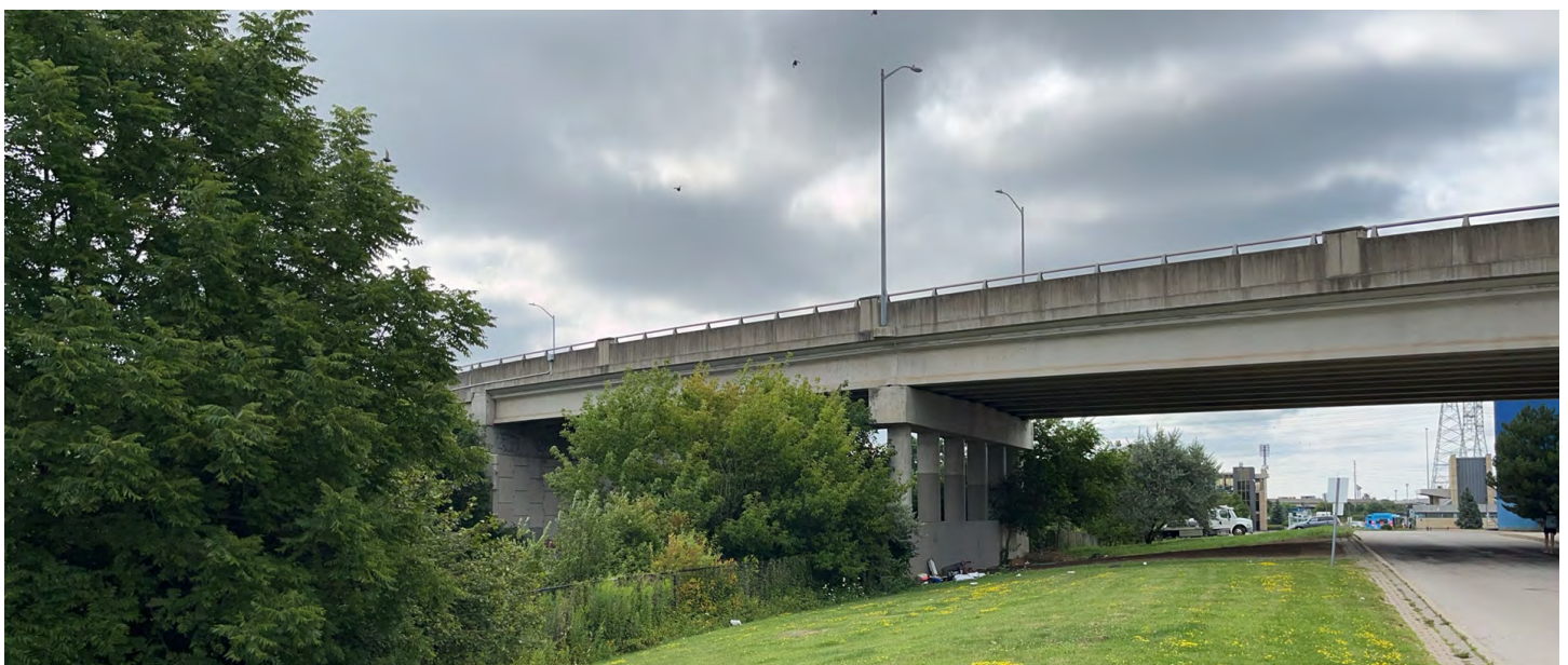
High Tech Road Bridge
