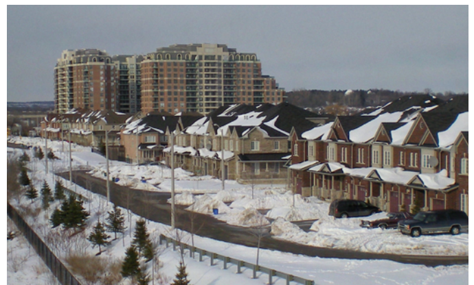
RESIDENTIAL DEVELOPMENT IN THE CENTRE TODAY
