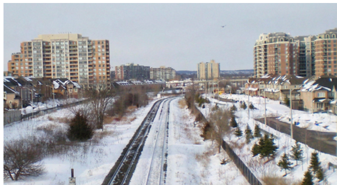
CN RAIL CORRIDOR
